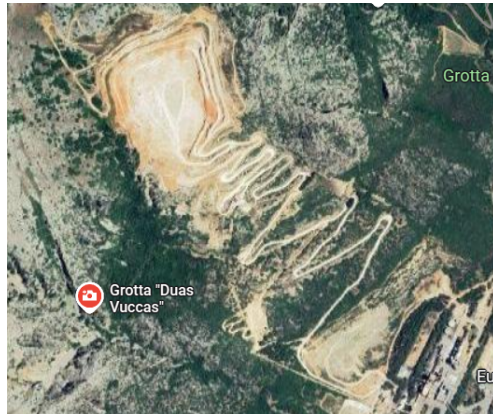
Aerial photo of the excavations of the UNICEM, a cement factory in Siniscola
